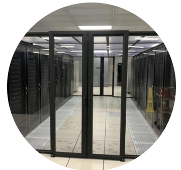
Cold Aisle Containment
